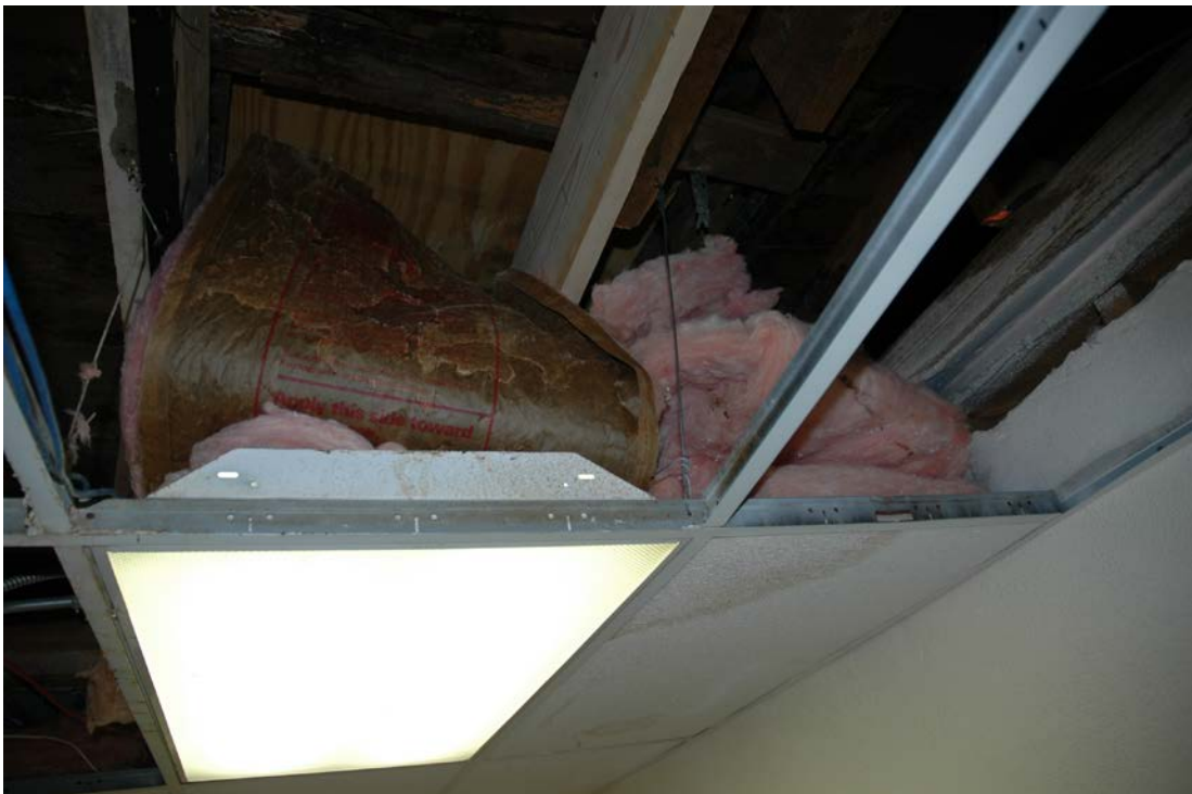
Ceiling Damage due to Water Leak
