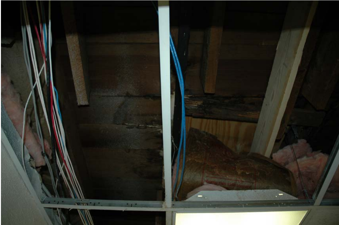
Ceiling Damage due to Water Leak
